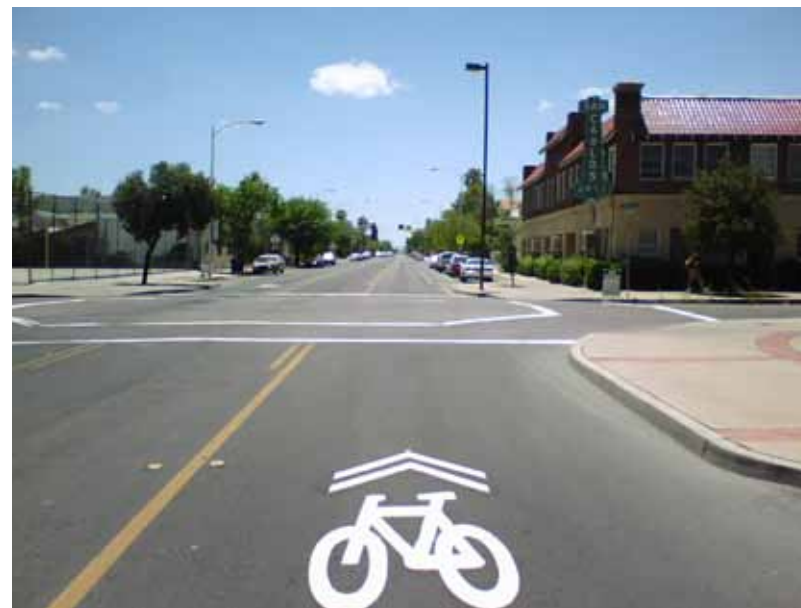
Sharrow pavement marking
